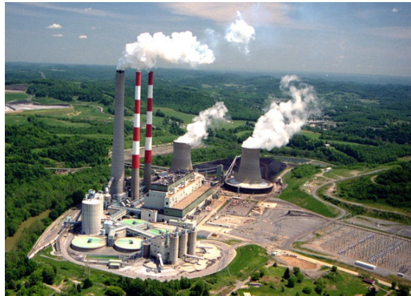
The 2-GW coal-fired Harrison Power Station | FirstEnergy
